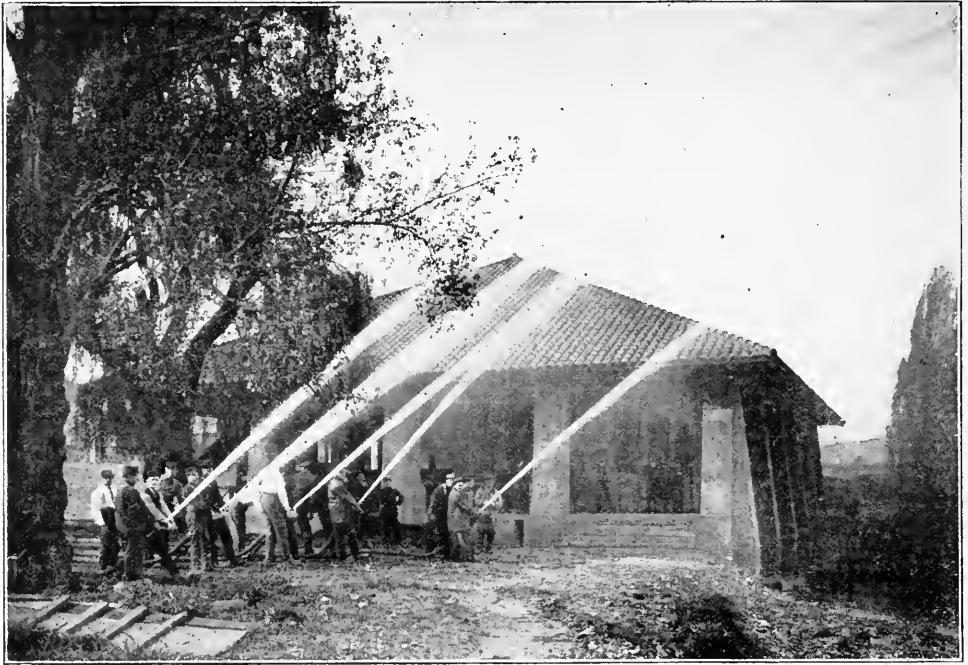
Pumping Station near Lake Merritt
